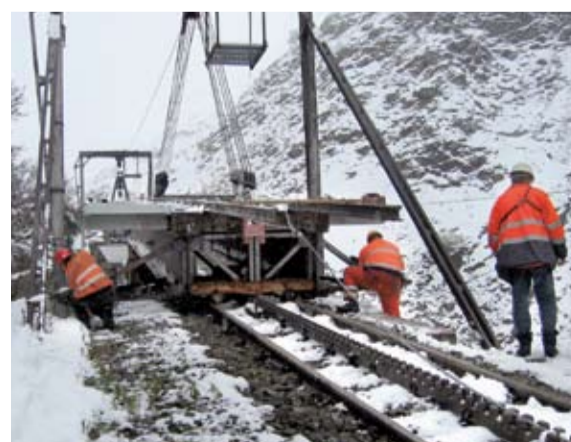
During dismantling and re-erection of the bridge, the HK winches are positioned on the track (left) and then pull the several-tonne bridge sections into place (right).
