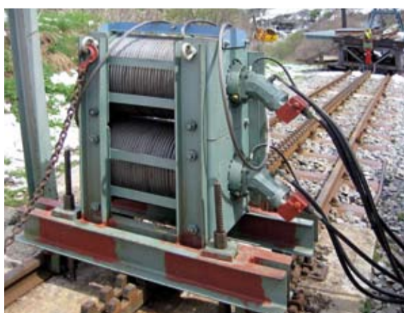
During dismantling and re-erection of the bridge, the HK winches are positioned on the track (left) and then pull the several-tonne bridge sections into place (right).
