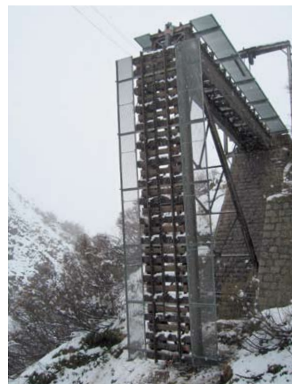
The Steffenbach bridge is "folded up" during the winter months due to the danger of avalanches.
