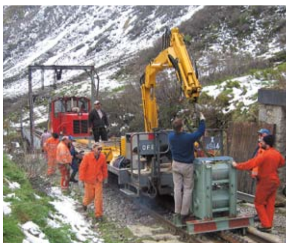
Rotzler HK 075 winches in use for dismantling the bridge.
